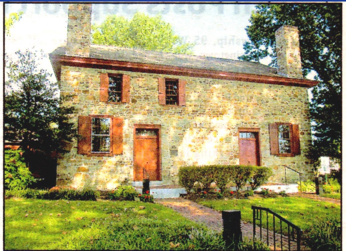
The Uwchlan Meeting House, located at 5 N. Village Ave., Lionville, was placed on the National Register of Historic Places in 1973.
