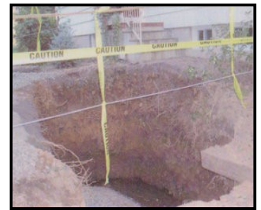
Hole in front yard
